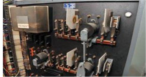
Electrical switchboard with asbestos flash guards. Switchboards can also contain an A-C sheet or resin/black backboard that contains asbestos. (non-friable)
