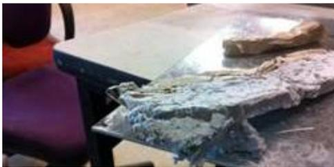
Mastic backed Asbestos fibre fire stopping around HVAC / other penetrations (friable)
