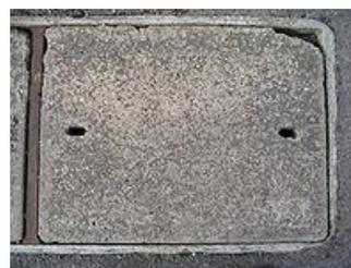
Telecommunications service pits were constructed using asbestos. Note the broken corner with potential for exposed fibres.
