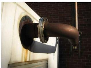
Asbestos gaskets in pipe flange joints (non-friable unless disturbed)
