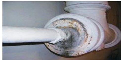
Amosite and chrysotile packing on a water pipe (friable)
