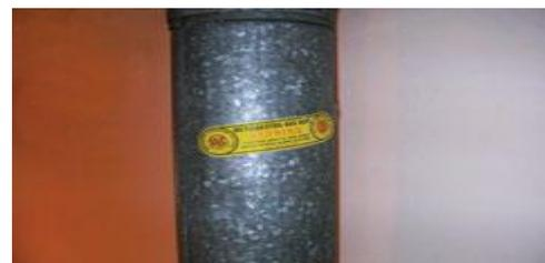
Metal clad gas Flue containing chrysotile lining (non-friable)
