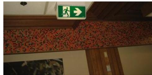
Ceramic tiles laid over a.c Sheet (chrysotile) backing (non-friable)
