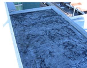
Asbestos reinforced bitument floor membranes (non-friable).
