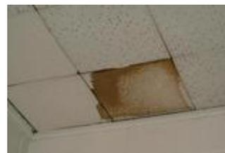
Asbestos containing ceiling tiles (non-friable unless damaged)
