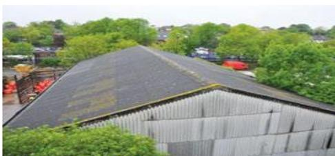
A-C roof and wall cladding (non-friable)
