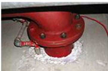
Fire stopping around floor penetrations (non-friable unless damaged or loose)
